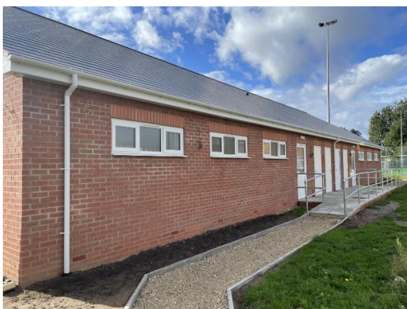
New PE Changing Rooms opening after half term
